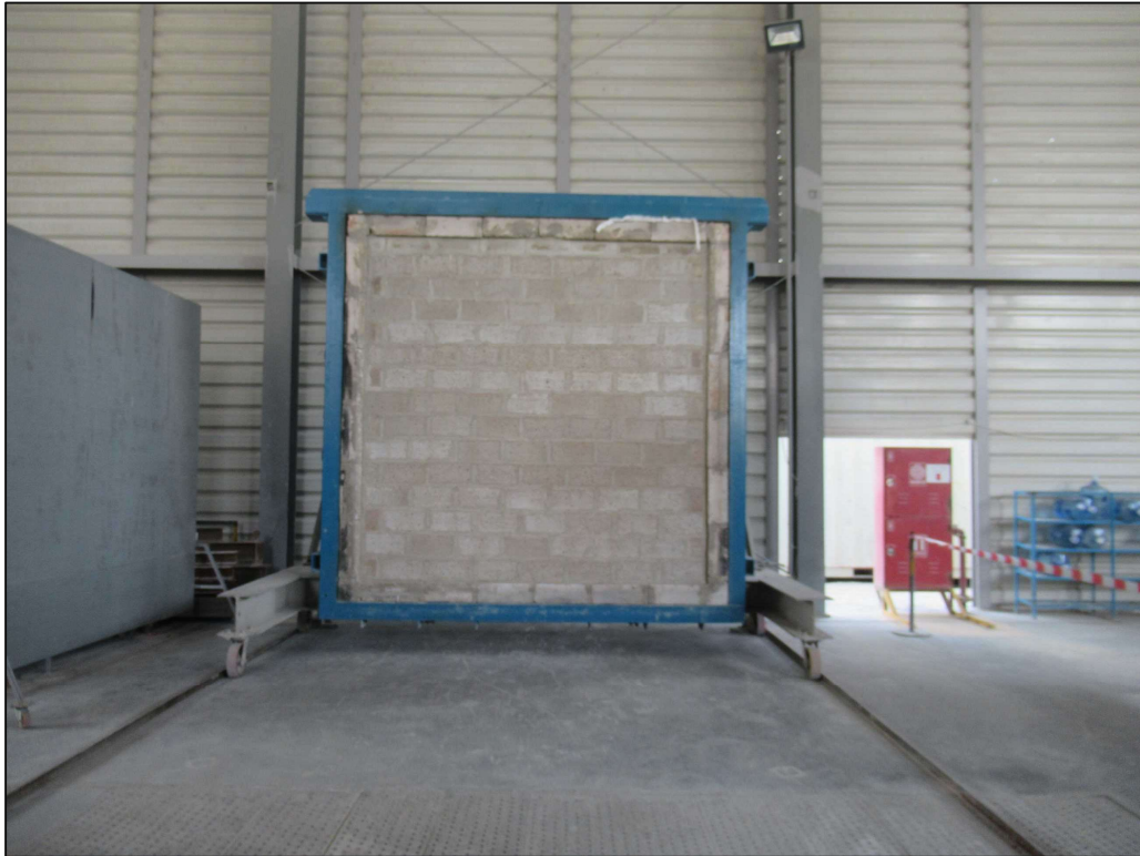
Picture 13: The exposed face of the specimen prior to the start of the hose stream test.
