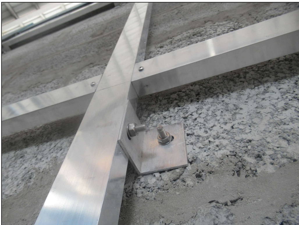
Picture 2: The horizontal runners connected to the vertical runners.
