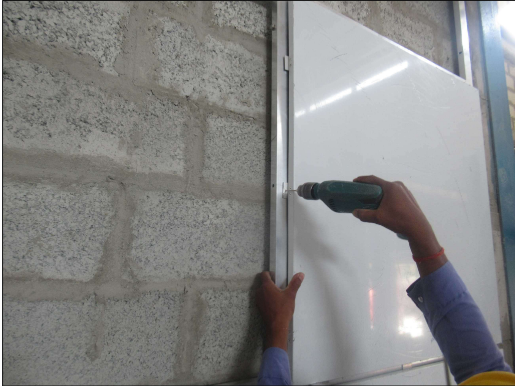
Picture 5: The ACP being fastened to the runners.
