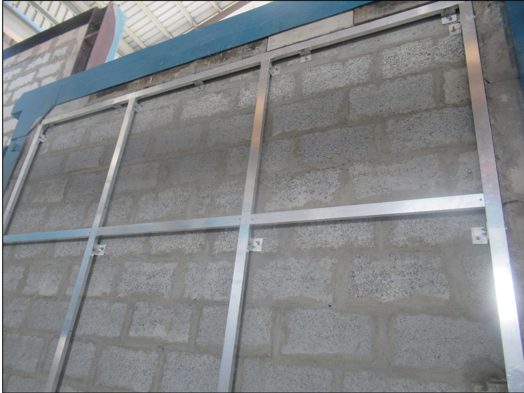
Picture 3: The specimen after the framing system was completely installed.
