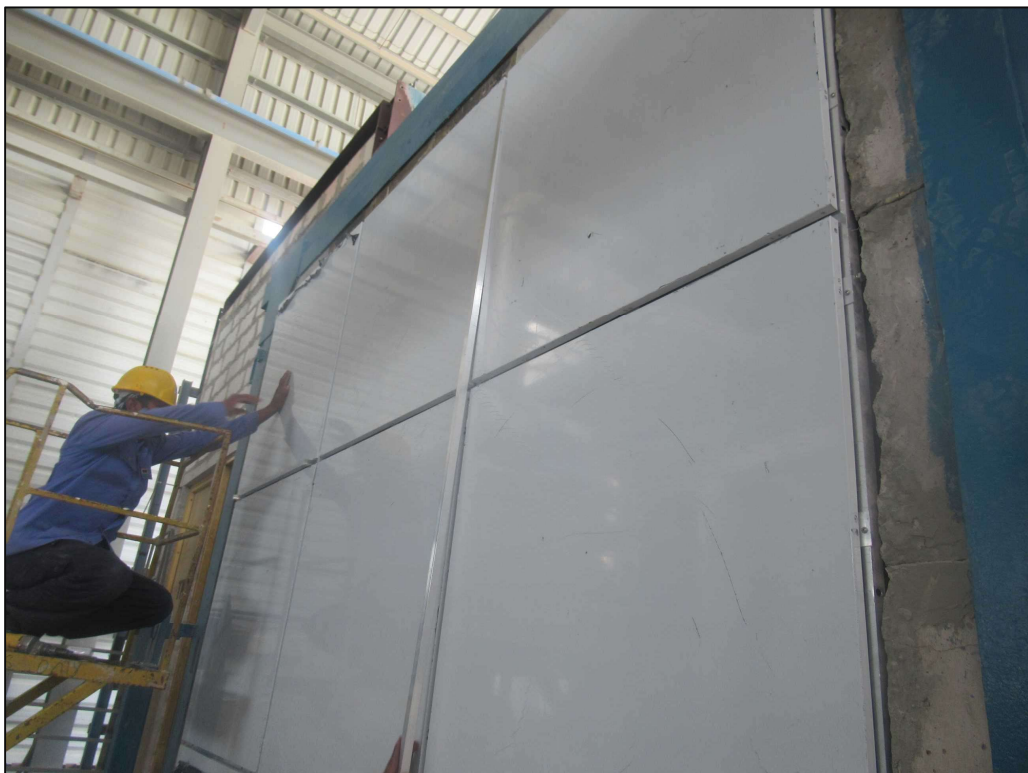
Picture 6: The U-channels being fixed to the panel gaps.
