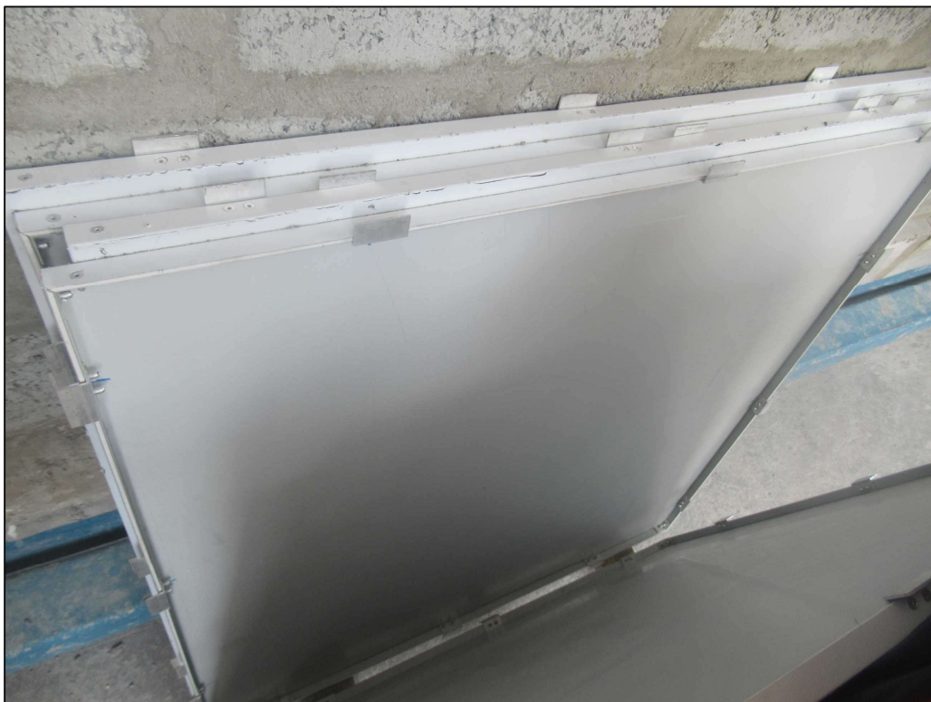
Picture 4: The tray profile of the ACPs.
