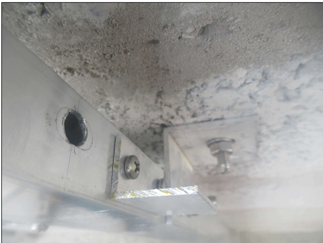
Picture 2: The connector fastened to the vertical runner.
