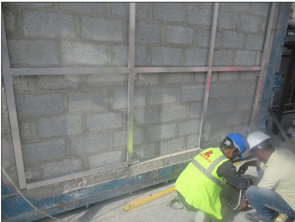
Picture 4: The specimen after the framing system was complete.
