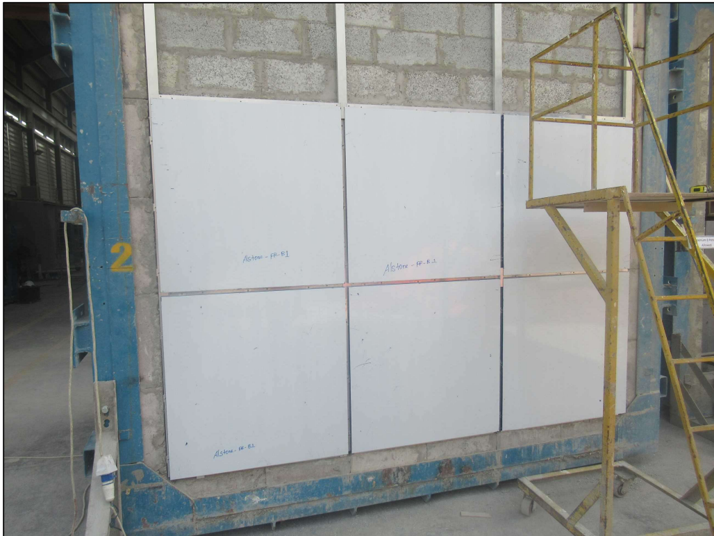
Picture 5: The ACPs fastened to the framing system.
